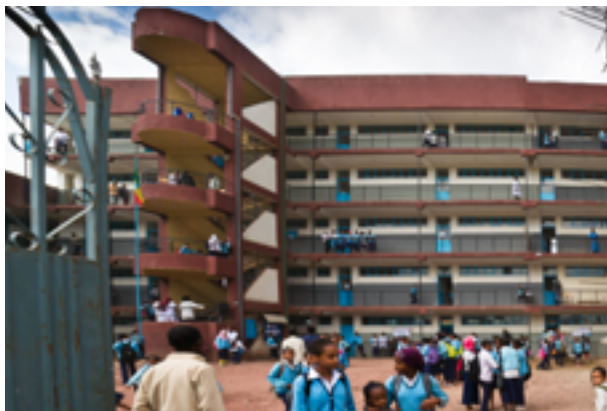
Future Generation Hope Secondary and Primary School Addis Ababa
